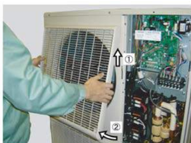
Remove the FAN GUARD by sliding upward.
