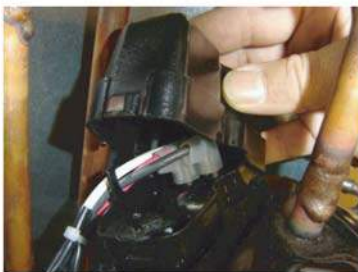
Remove the TERMINAL COVER.
