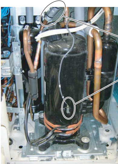
Discharge temp. thermistor (TH1)
