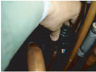
Remove the EEV coil by hand. There are two coils.
