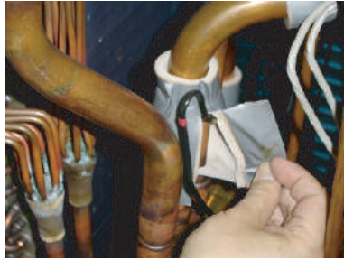
Remove the heat insulation.
