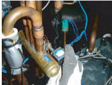
Remove the SOLENOID COIL.
