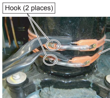
Crank Case Heater (2 places)
