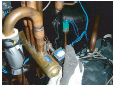
Remove the SOLENOID COIL.
