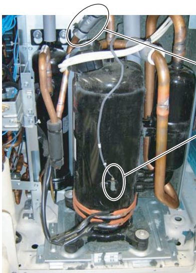
Discharge temp. thermistor (TH1)
