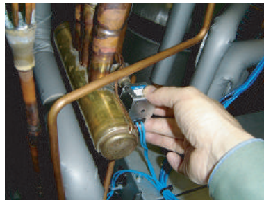
Remove the SOLENOID COIL.
