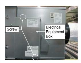
1: First remove the screw (2 pieces) and then remove the cover of Electrical Equipment Box.
