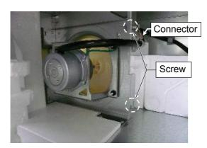
4: Turn two pieces of screw on the Motor ASSY and remove the wired connector.
