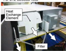
3: Remove the Heat Exchange Element and the filter.
