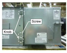
2: Turn the knob (2 pieces) and the screw (1 piece) and remove the Inspection Cover.
