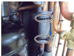
Thermistor (Discharge)
