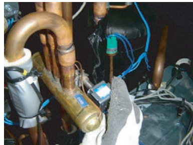
Remove the SOLENOID COIL.
