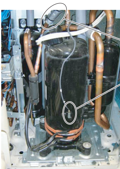
Discharge temp. thermistor (TH1)
