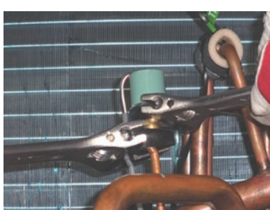
Remove the PRESSURE SENSOR with wrench. There are two sensors. (High and Low pressure) Note the tightening torque at the installation. Tightening torque is 15 \pm 1.5 \text{ N}\cdot\text{m} .
