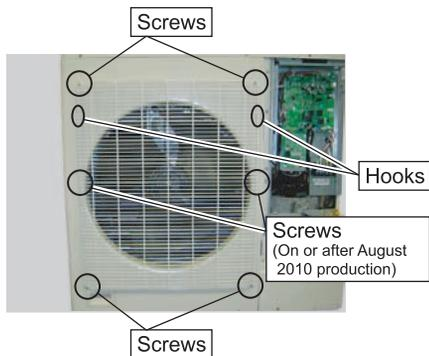
Remove the 4 mounting screws.
