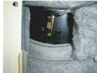
Remove the THERMISTOR SPRING
