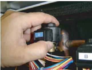
Remove the EEV coil by hand.
