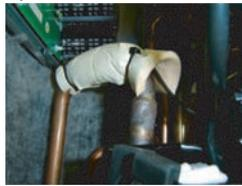
Cut the binder, and remove the heat insulation.
