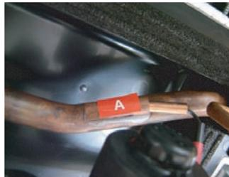
Remove the THERMISTOR SPRING. Remove the THERMISTOR.
