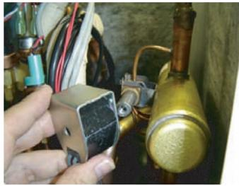
Remove the SOLENOID COIL.
