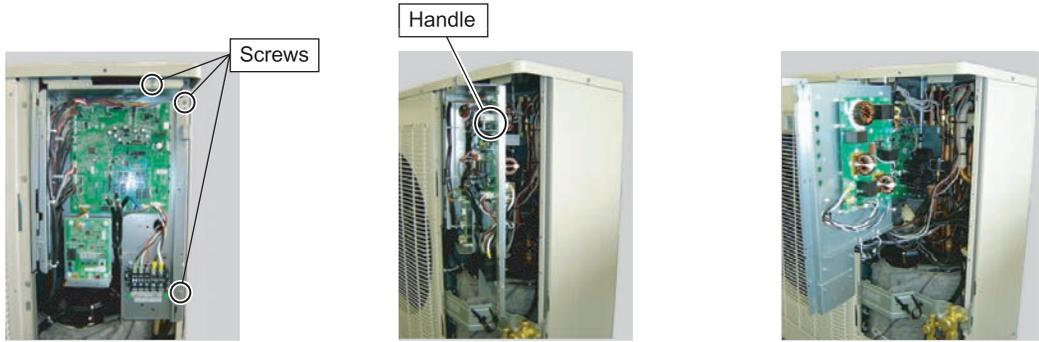
Remove the 3 mounting screws.
