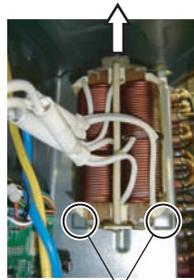
Remove the COIL CHOKE by sliding upward.
