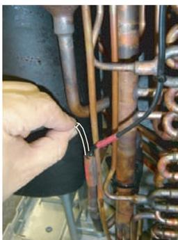
Remove the THERMISTOR SPRING.
